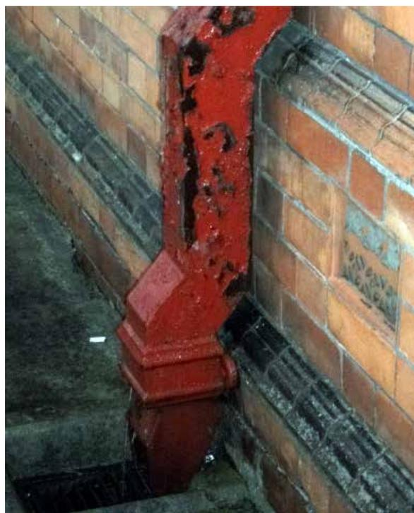
**Cast Iron Rainwater left unprotected: the gutter is painted in red primer only**
